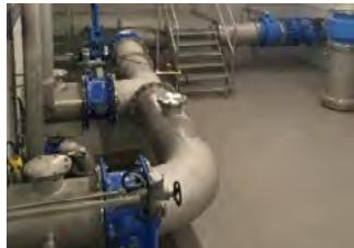
ERHARD Butterfly Valves are installed in large, medium and small scale hydropower plants and dams, mostly designed as safety valves for over-speed protection and main pipe burst control, suitable for up to 30 m/s flow velocity.
