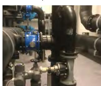
In water treatment plants, the inside of the valve is protected with enamel coating against salt water, limescale and abrasion by sand or other hard elements, and is thus also suitable for brackish and seawater.
